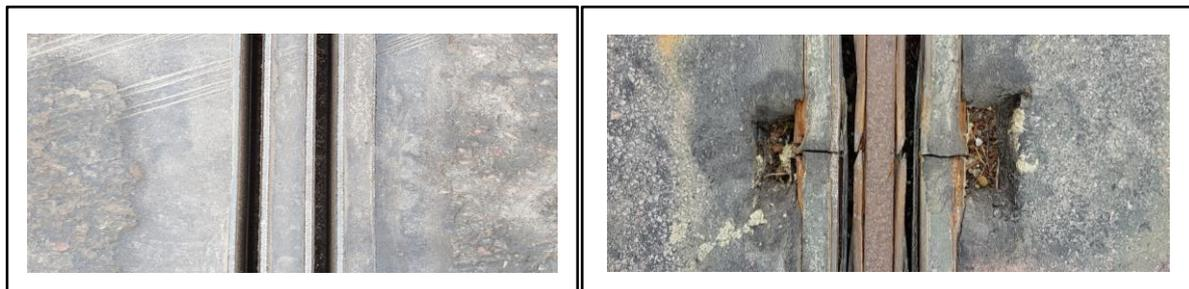
*Figure 1: Example of a conductive rail ERS solution with perfect alignment with the road surface in the first picture and a more worn-down pre-demonstration test solution in the second picture. Photo: Lina Nordin and Terence McGarvey.*
